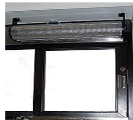
Air curtain over pass through window
